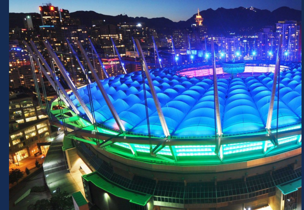
BC PLACE STADIUM, VANCOUVER, CANADA
