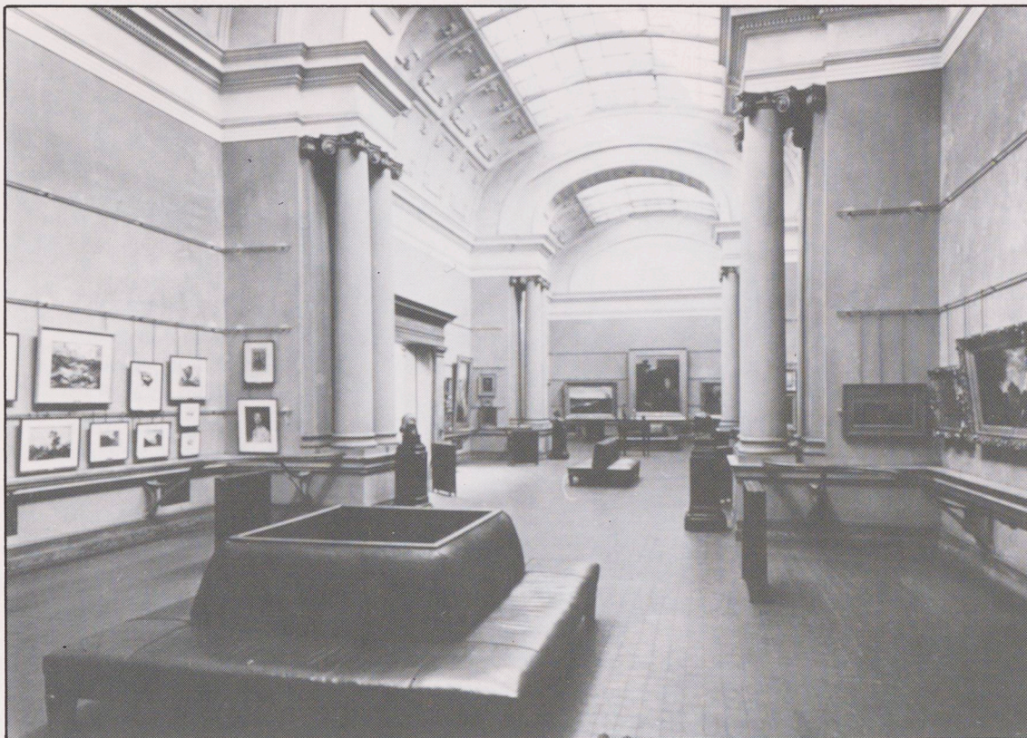
The Mackelvie Gallery, about 1950, immediately before its transformation
